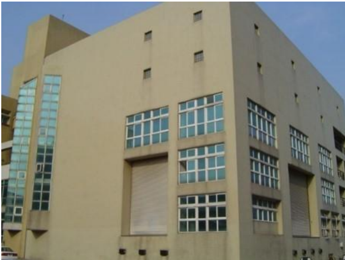
Exterior View of the Large Cavitation Tunnel Facility
