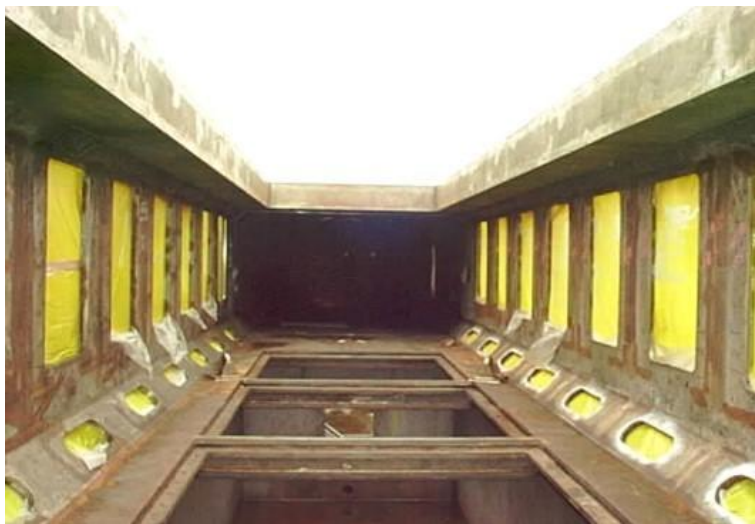
Test Section of the Large Cavitation Channel
